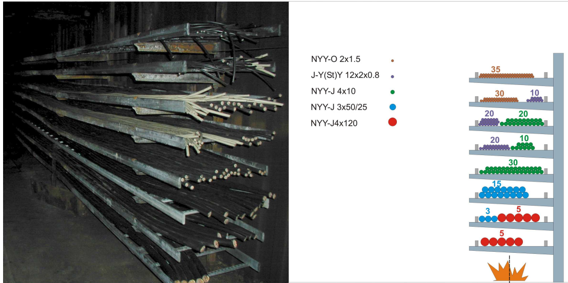
Figure 1 Left: photograph of the cable tray fuel package; right: schematic illustration of the cable arrangement
