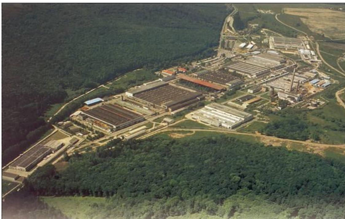
Figure 8. Mechanical industry plant of PPS Group Inc. at Detva, Slovakia. Source: ECB/PPS Group
