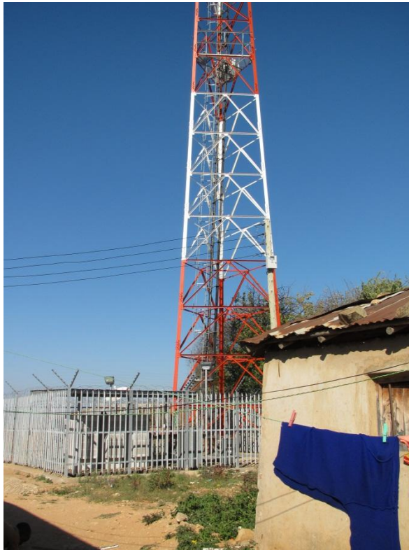
Figure 11. Mwangata base-station tower.
