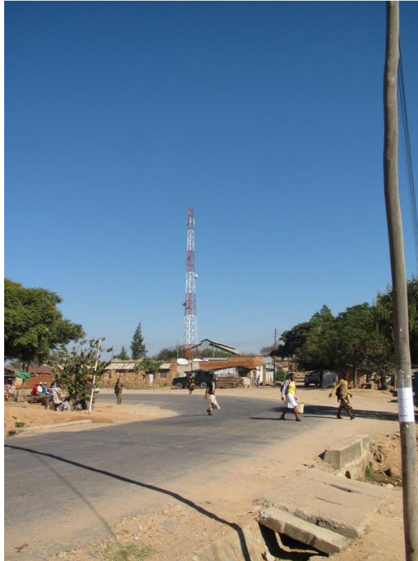
Figure 12. Mwangata base-station tower.
